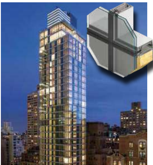
LEXINGTON AVENUE Lokalisatie: New York / USA Project: Time Square Development
