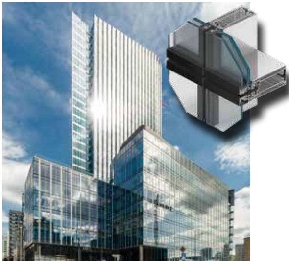
MENNICA LEGACY TOWER Lokalisatie: Warsaw Project: Goettsch Partners
